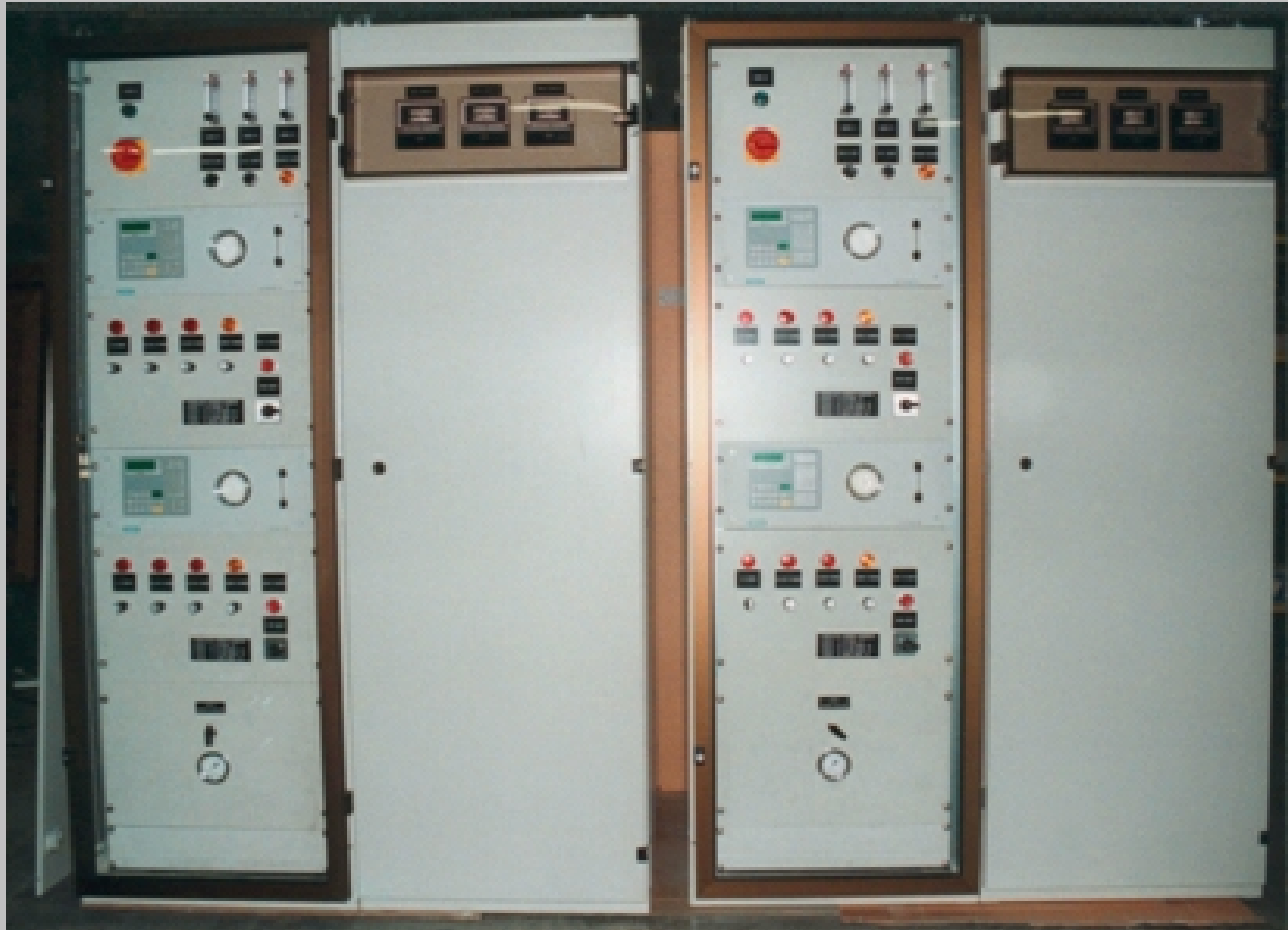
Power Plant - Gas Monitoring Systems
